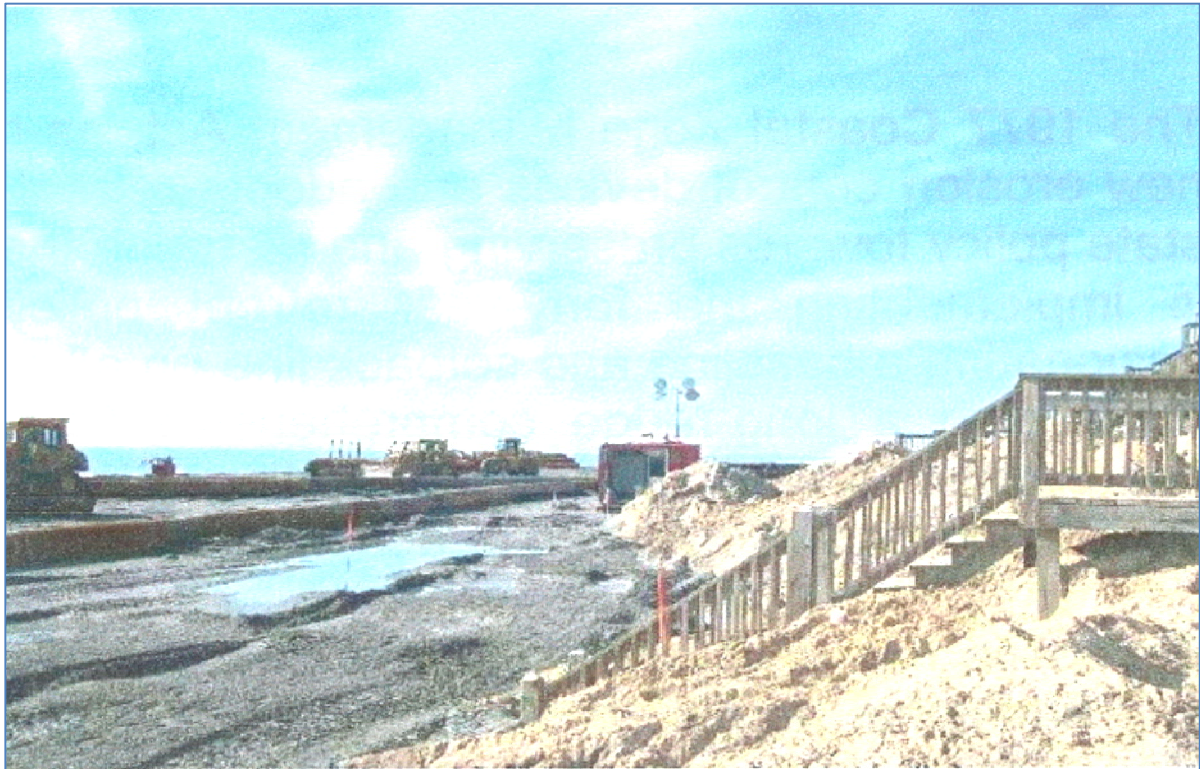
Photo 23. Beach renourishment project occurring in North Myrtle Beach in 2008.
