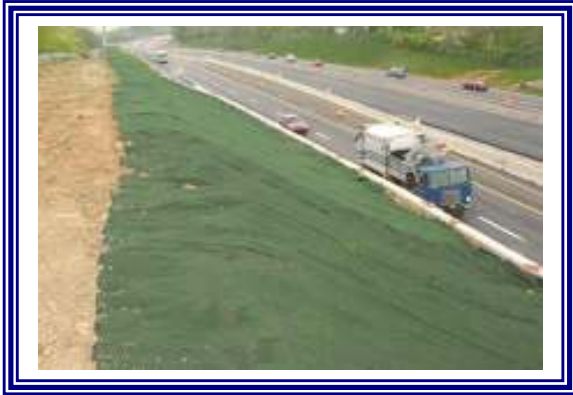
TRM Slope Application
