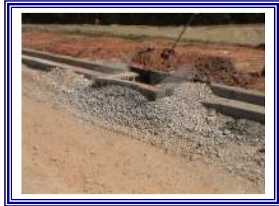
Block and Gravel Inlet Protection
