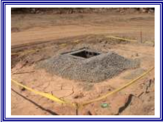
Block and Gravel Inlet Protection
