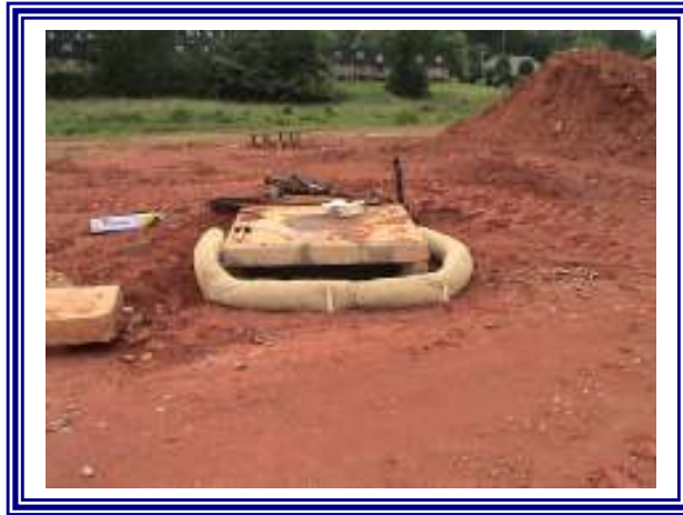
Sediment Tube Inlet Protection
