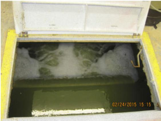
Photo 2: Discharge over 5-foot rectangular weir
