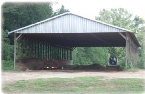
Compost sheds were built to keep litter covered and dry before application.
