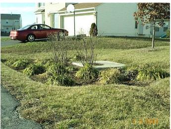
Figure 2. Drop Inlet Structure Located in Bioretention Area
