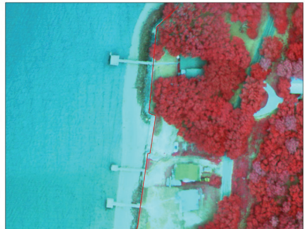
Vertical Structure fronted by Sloped Structure (101.1)
