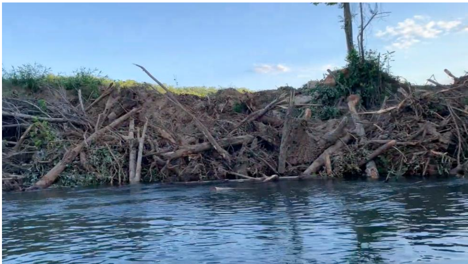
Photo 24. Woody debris dumped along erosional reach of the South Saluda River
