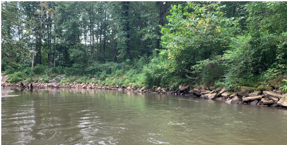
Photo 22. Rock Toe Bank stabilization on the South Saluda River
