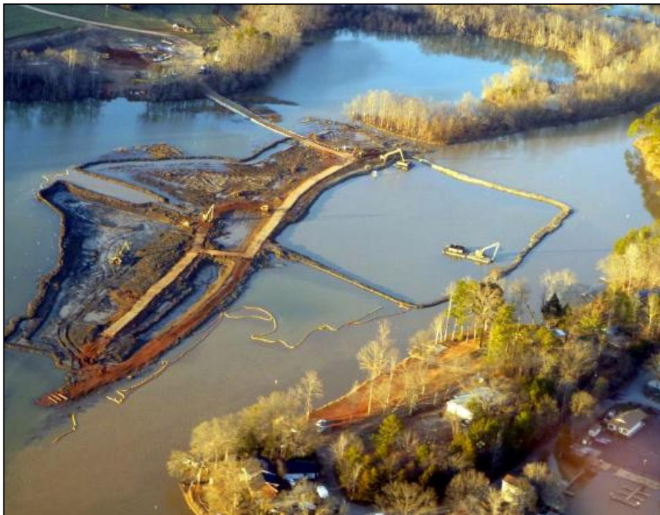
Photo 5. Saluda Lake dredging operation, 2012
