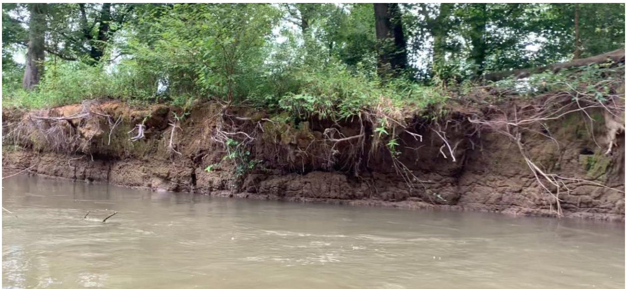
Photo 20. Eroding riverbank on the South Saluda River
