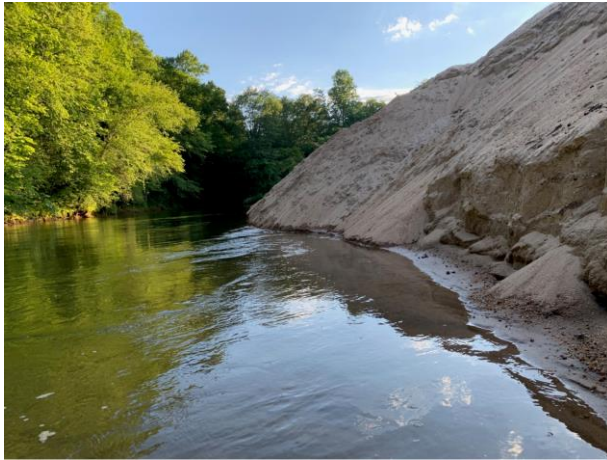
Photos 26 and 27. Unstable riverbanks near sand dredging operation
