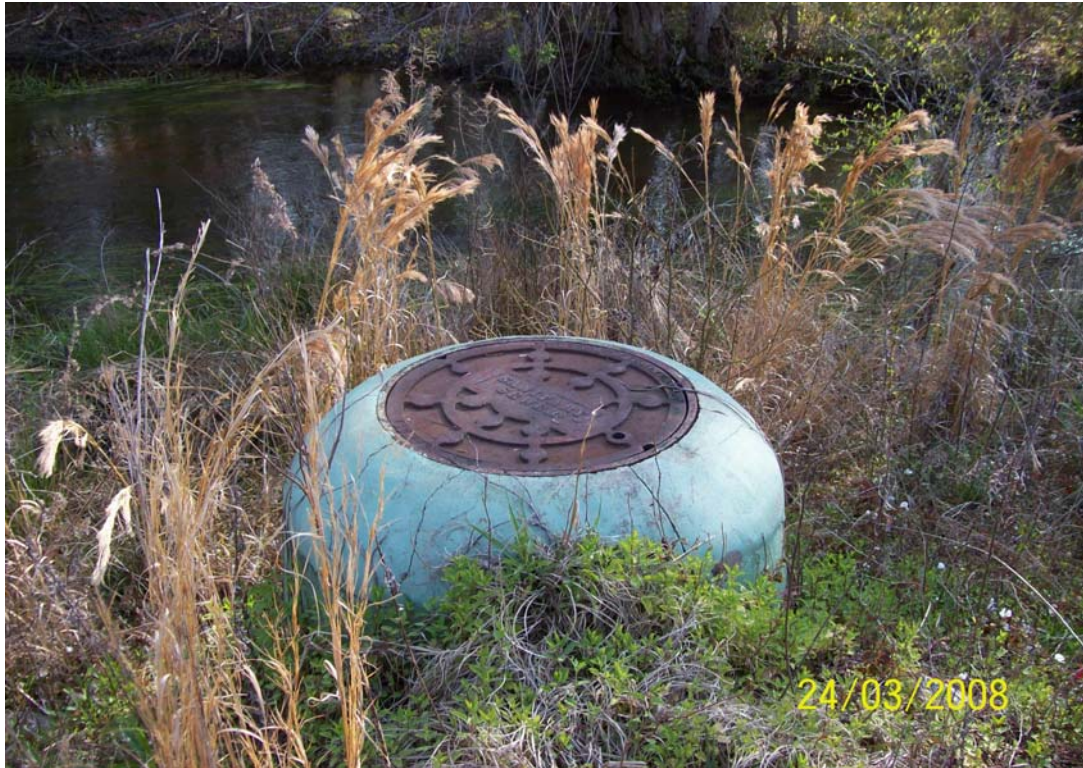
Sewer located along the banks of impaired station E-105
