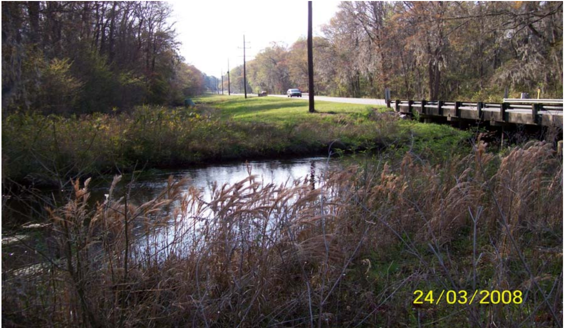
Bridge crossing over impaired station E-105
