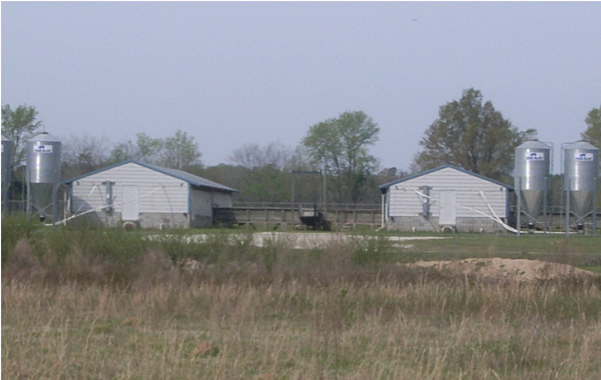
Figure A-3. Patterson Swine Facility
