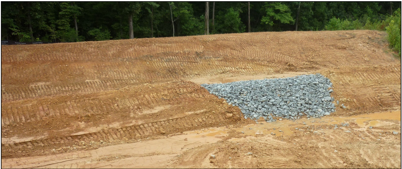
Photo: Sediment Forebay
