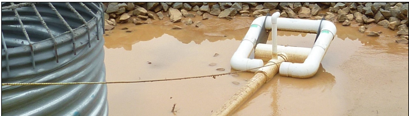
Photo: Skimmer with Attached Rope for Ease of Maintenance
