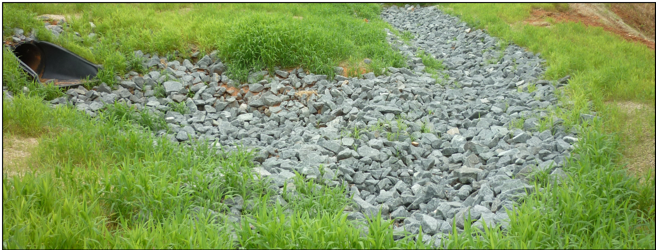
Photo: Principle Spillway's Barrel (Outlet Pipe) with Plunge Pool and Level Spreader
