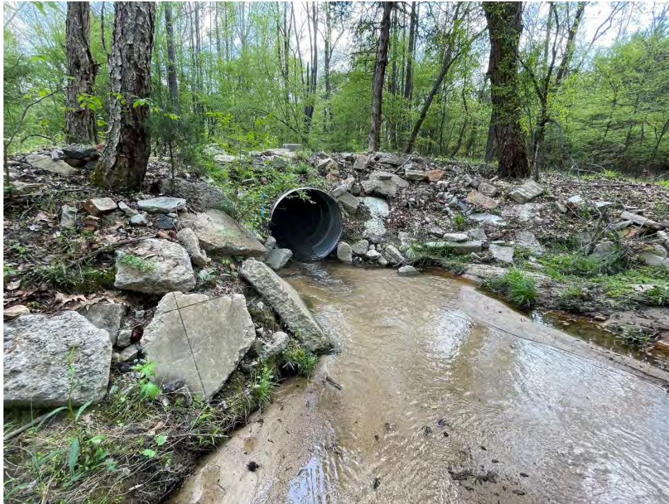
PHOTO 27: Culvert Associated With Non-Wetland Water STA (Perennial) Road Crossing
