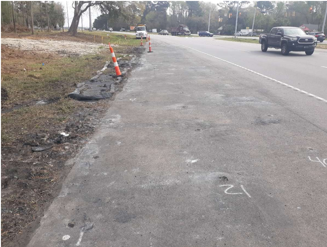
Shoulder work zone restoration – March 22, 2022
