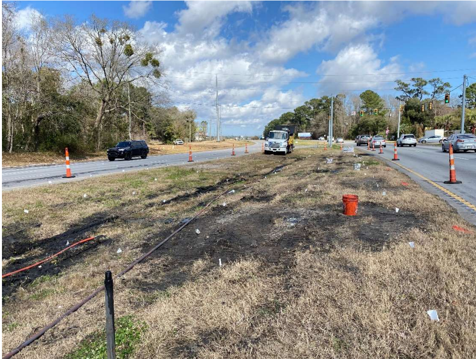
Injection grid layout in median – February 18, 2022
