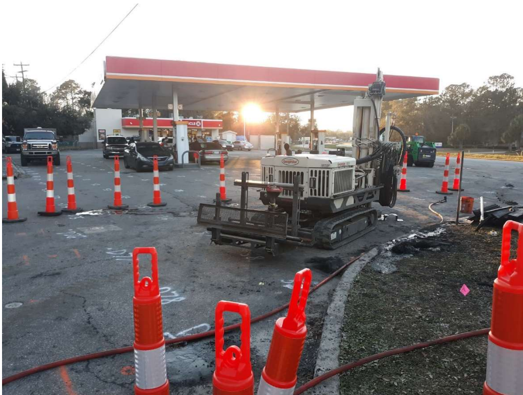
On site injection area – January 18, 2022
