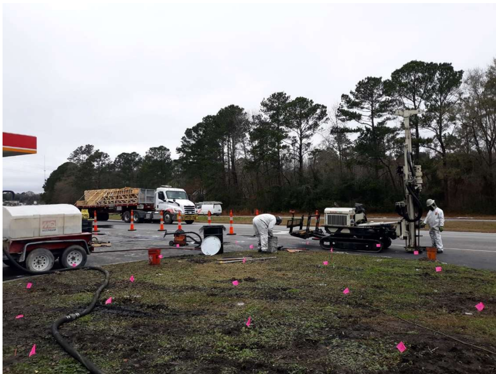
Injecting point B-57 – January 21, 2022
