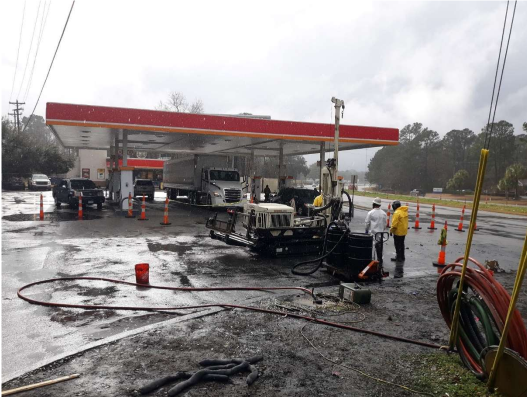
Injecting in Area A – February 16, 2022
