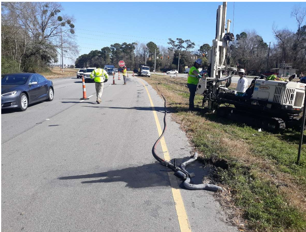
Daylighting while injecting C-03 – February 19, 2022
