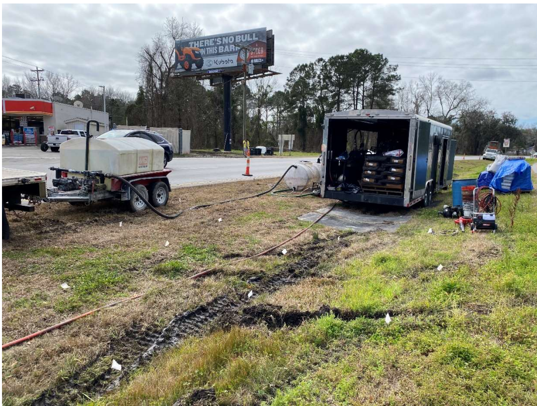
Injection system setup in median of US-17 – February 17, 2022
