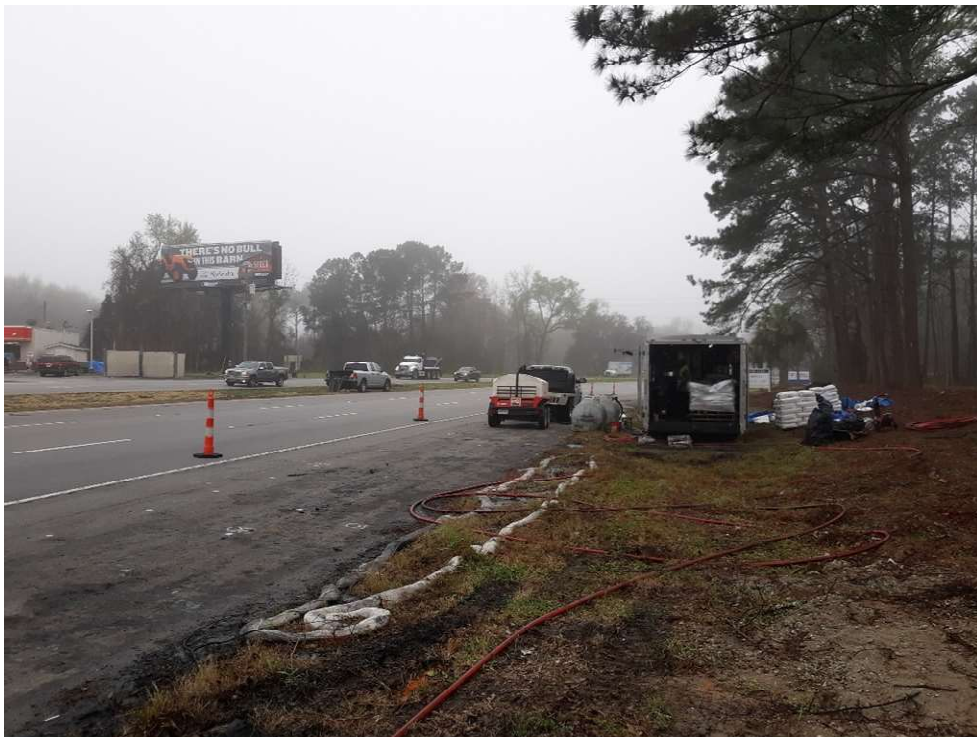
Injection system setup on southbound shoulder of US-17 – March 17, 2022
