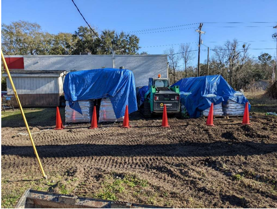
Injection materials staged and secured – January 12, 2022
