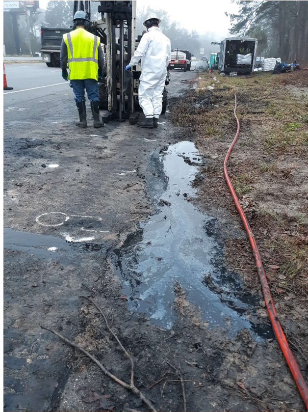
Daylighting while injecting F-20 – March 17, 2022
