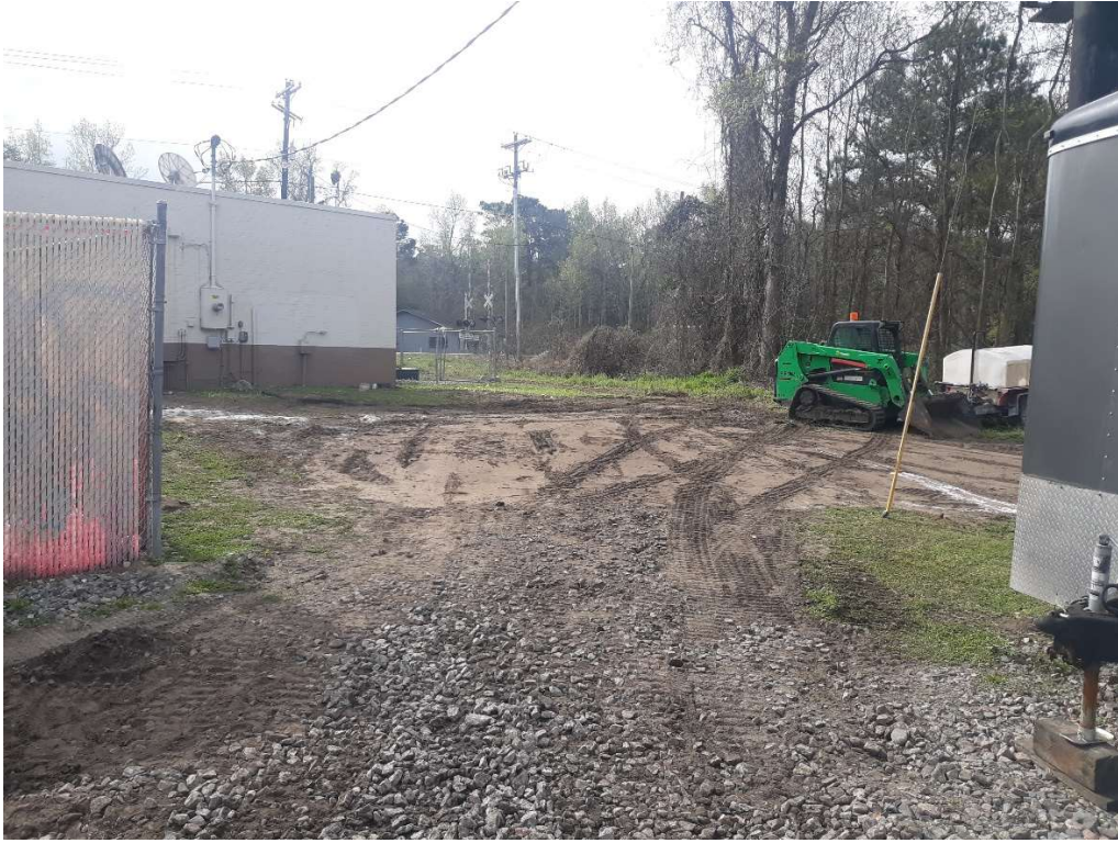
Material staging area restoration – March 22, 2022
