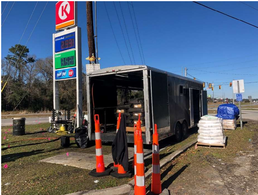
Injection system setup on site – January 18, 2022
