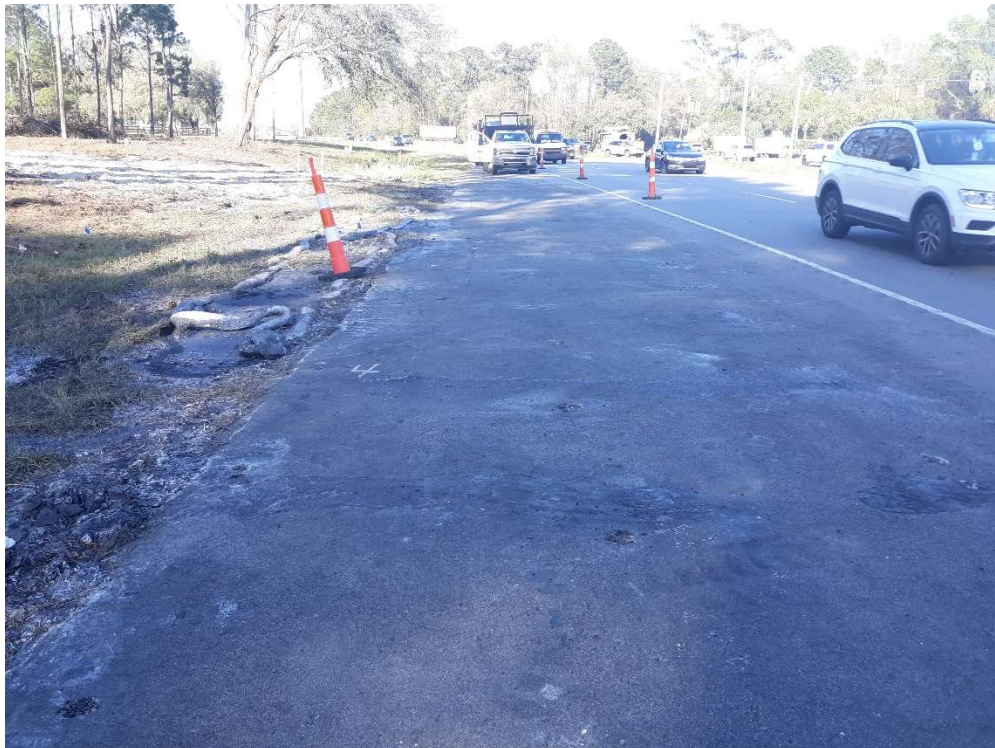
Shoulder work zone restoration – March 21, 2022
