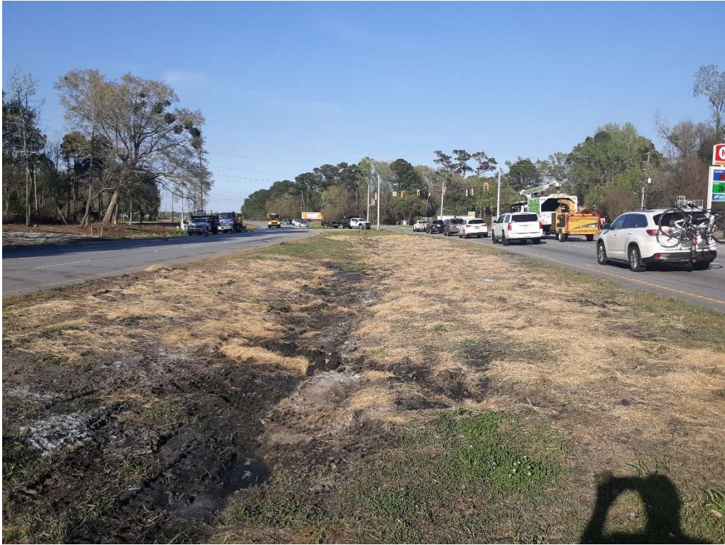
Median restoration – March 17, 2022
