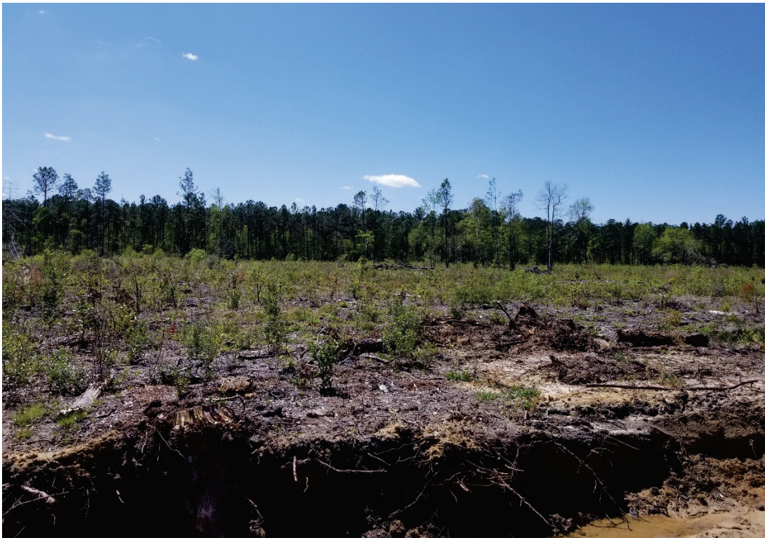
Figure 4. General views showing project location. Upper photo shows the access road and ditching. Lower photo shows the clear cutting and general ground condition.
