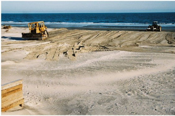
FIGURE 2.10. Photos of the 2004-2005 sand scraping and transfer project. [UPPER LEFT] Pan earthmovers loading sand from North Beach at low tide. [UPPER RIGHT] A bulldozer and farm tractor with scraper blade grading and dressing the beach. [LOWER LEFT] Regrading and dressing slopes around Oystercatcher beach access. [LOWER RIGHT] Scraped sand in place against the seawall around Beach
