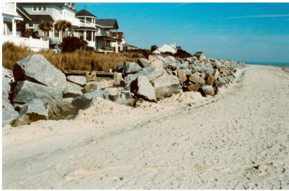
FIGURE 2.10. Photos of the 2004-2005 sand scraping and transfer project. [UPPER LEFT] Pan earthmovers loading sand from North Beach at low tide. [UPPER RIGHT] A bulldozer and farm tractor with scraper blade grading and dressing the beach. [LOWER LEFT] Regrading and dressing slopes around Oystercatcher beach access. [LOWER RIGHT] Scraped sand in place against the seawall around Beach
