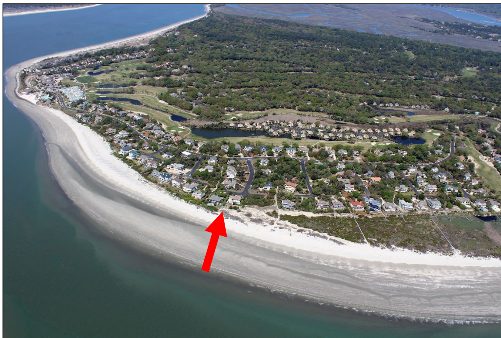
FIGURE 3.5. Reaches 4, 5, and 6 along Seabrook Island are armored by a quarry stone seawall that is now buried by sand transported south from Capt Sams Inlet by natural, as well as, artificial means. Arrow marks the location of Fig 3.4 where the 1970s seawall has been completely buried under a vegetated dune. [Image by SB Traynum – CSE on 11 April 2018]
