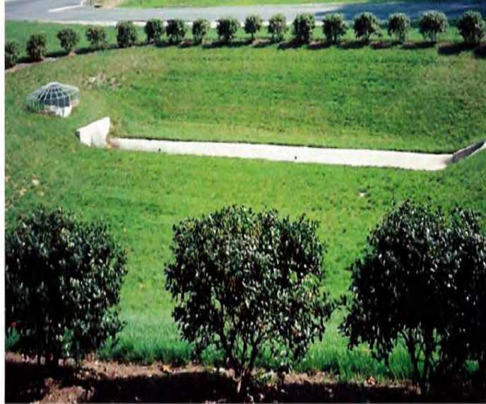
Figure 4-2: Detention (Dry) Pond
