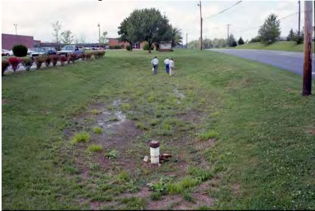
Figure 4-13: Perimeter Sand Filter
