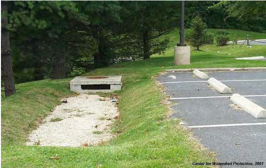
Figure 4-10: Infiltration Trench
