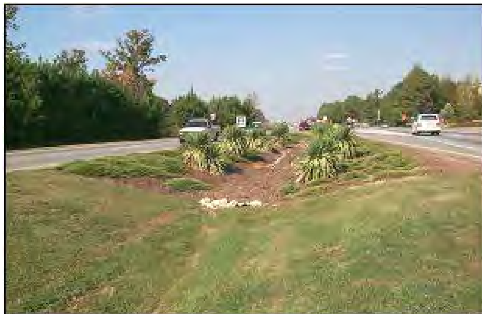
Figure 4-20: Enhanced Dry Swale
