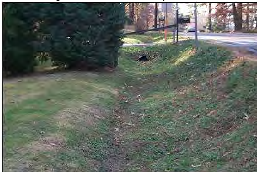
Figure 4-15: Grass-Lined Open Channel
