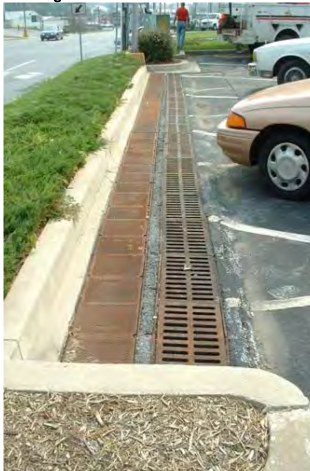
Figure 4-13: Perimeter Sand Filter
