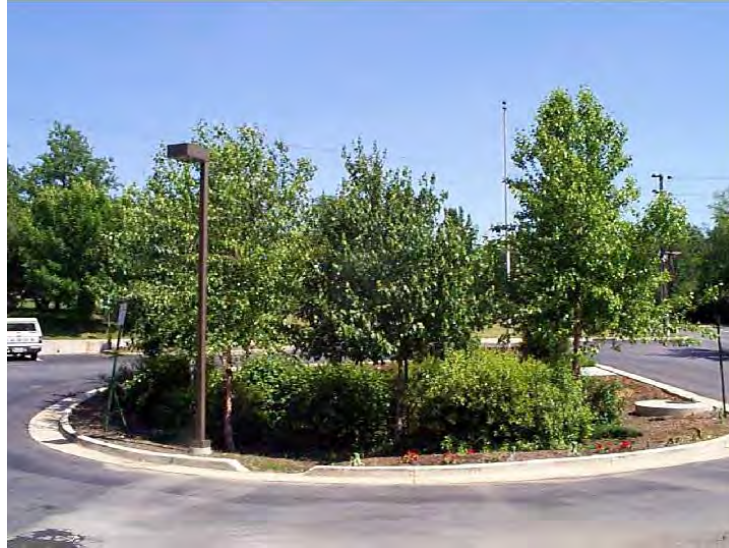
Figure 4-8: Bioretention in a Parking Lot Turnaround
