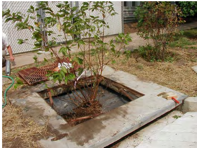
Figure 4-22: Tree Box Filter
