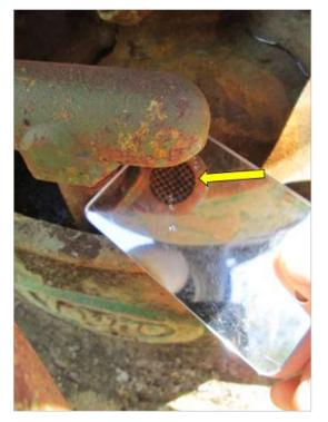
FIGURE 5. East Voorhees well vent (well vent with screen mesh larger than #24).
