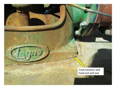
FIGURE 6. East Voorhees well mounting (crack shown between well head and pad).
