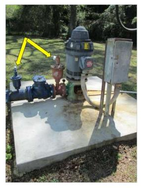
FIGURE 4. East Voorhees well head and pad (casing does not extend 12 inches above pad and air relief valve discharge is not downturned and screened).
