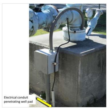
FIGURE 7. Acacia well site (electrical conduit shown penetrating well pad).
