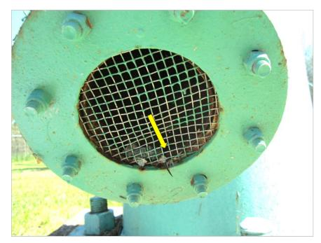
FIGURE 18. East Voorhees storage tank overflow showing trapped bird feathers.
